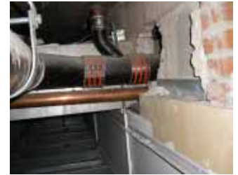
Example: 2-hour firewall penetration
