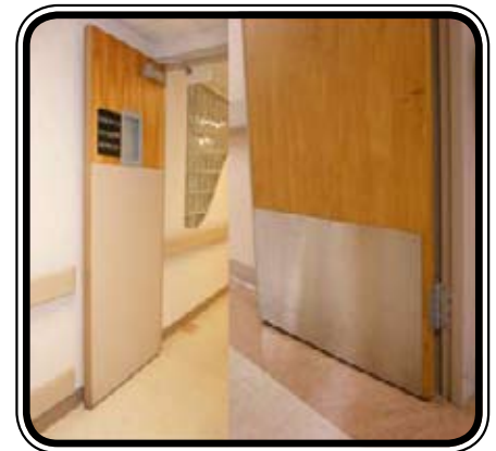
Pictured left is a door with a protective plate at 55 inches above the bottom of the door.
