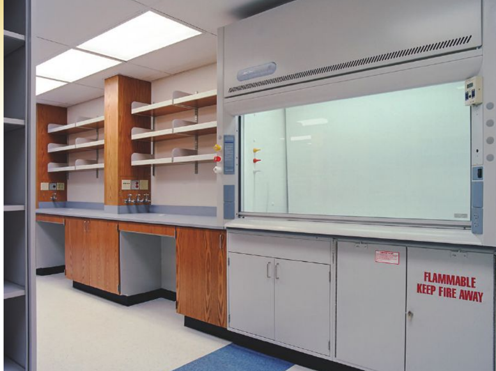
Figure 6: This shows a bypass fume hood recessed into the lab wall on top of a flammable storage cabinet with workspace adjacent. Notice the airflow velocity meter on the right of the hood.
