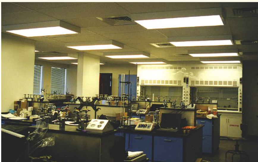
Figure 7: These lab work counters have two bypass fume hoods at the back wall. Notice the surface-mounted light fixtures indicating tight above-ceiling space.
