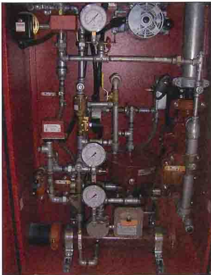
LEFT The inside of a preaction water-based sprinkler system cabinet, which is most often combined with a clean agent fire suppression system. RIGHT The interior of a power distribution unit with an isolation transformer.
