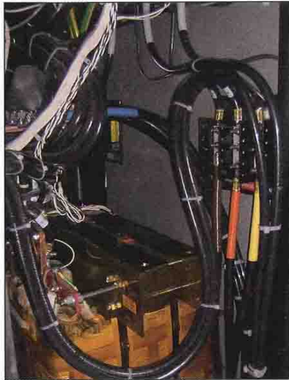
LEFT The inside of a preaction water-based sprinkler system cabinet, which is most often combined with a clean agent fire suppression system. RIGHT The interior of a power distribution unit with an isolation transformer.
