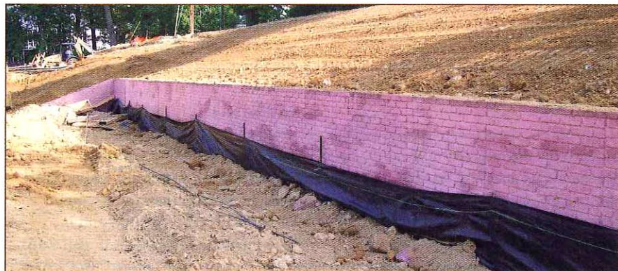
Retaining walls helped minimize the footprint of the CBU soccer field while maintaining the basin's required water retention level.
