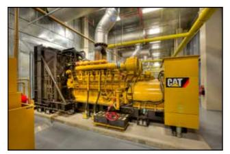
"A.8.4.1 Weekly inspection does not require running of the EPS. Running unloaded generators as part of this weekly inspection can result in long-term problems such as wet stacking. See Figure A.8.4.1(a) and Figure A.8.4.1(b)."
