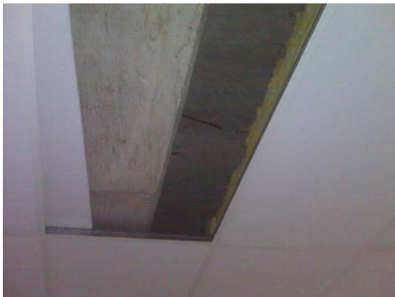
Figure 2. Insulation not present along column, but present in most of parking garage drop ceiling.
